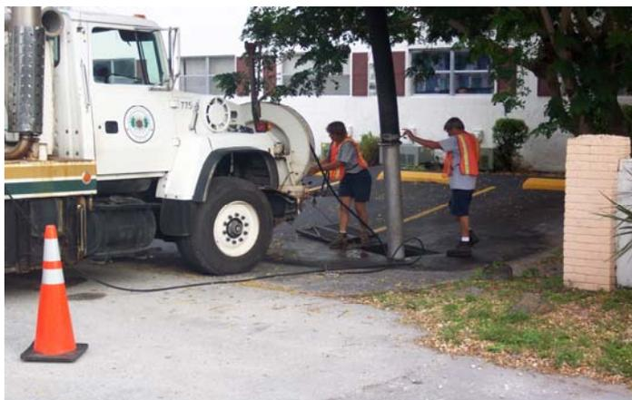
A: This is the Stormwater Division's VacCon—essentially a very powerful vacuum unit that sucks up debris from catch basins, storm drain lines, and sumps. The vacuum compressor produces 8,000 cfm (cubic feet per minute), a standard home vacuum cleaner produces about 85 cfm. The truck also has 600' of 1" hose, to which various nozzles are attached to propel the hose up lines and bring any debris back to the manhole or catch basin for suction and removal.
