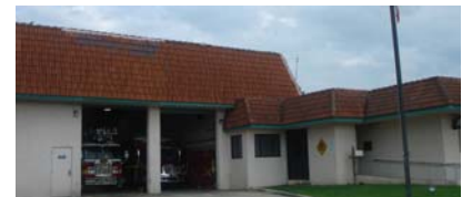
Station #87: 2100 NW 39th Street
