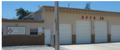
Station #20: 4721NW 9th Avenue
