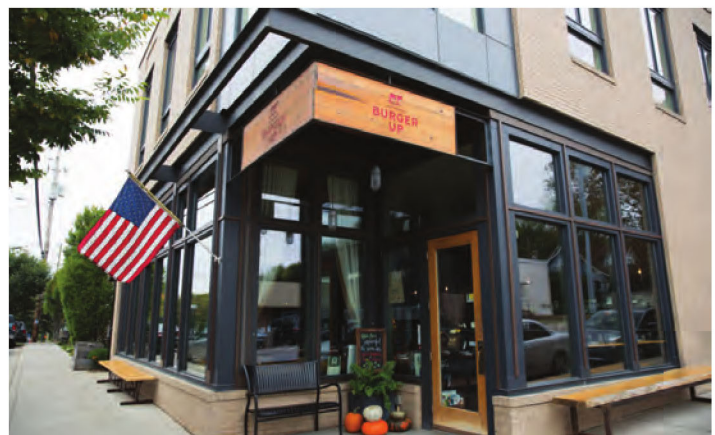
Carved entries create interior and exterior pedestrian visual interaction and provides covered outdoor areas.
