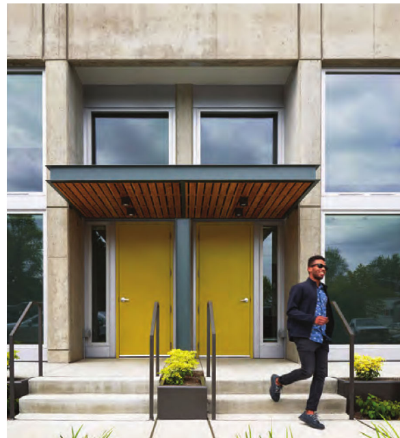
Canopies can help mark entries into buildings.
