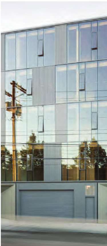
Locate service facilities within buildings, to the maximum extent feasible.
